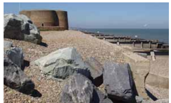
Coastal defences: the Martello Tower at Slaughden is protected by rock armour and groynes. The beach is regularly recharged by bulldozers.
