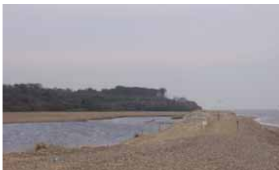
Easton Broad, showing the beach bar reinforced with bulldozed shingle, 2006. The eroding cliff at Easton Wood is in the background.
